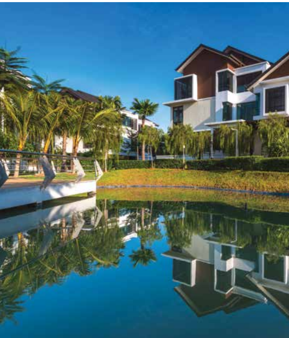
Rainwater Harvesting at Symphony Hills, Cyberjaya
